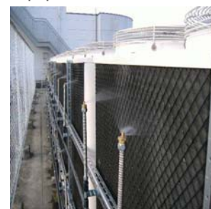
Outdoor equipment sprinkler system
