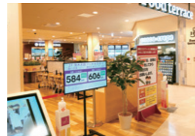
Introduced network-based CO 2 concentration monitoring system
